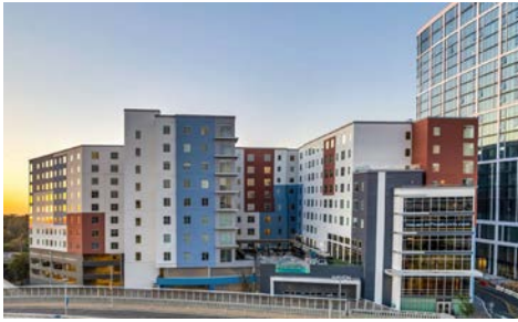
Haven 641 Division St | 299 Units
