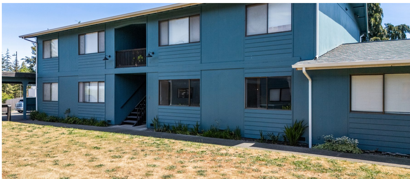
12-UNIT APARTMENT BUILDING — NEW ROOF INSTALLED 2024
