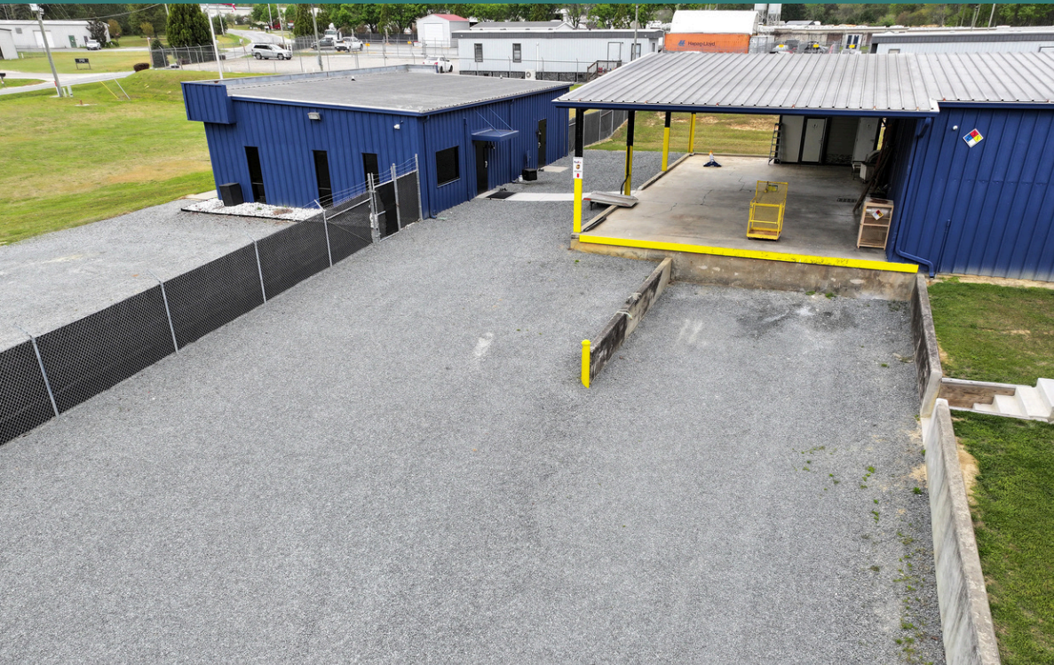
Dock Access & Office Building
