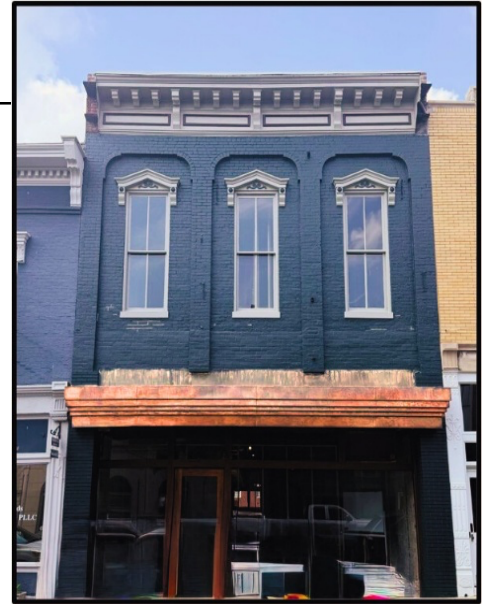
Photo: Exterior; Main Street
