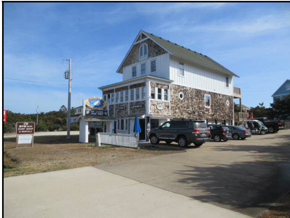
Subject View Facing Northeast
