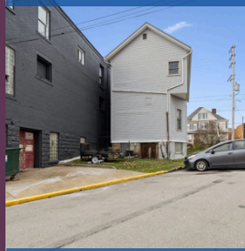
Back of Building
