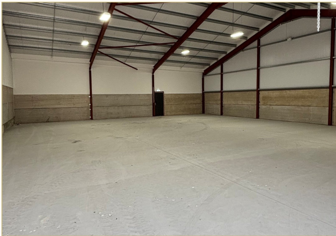
Interior — clear span, high eaves
