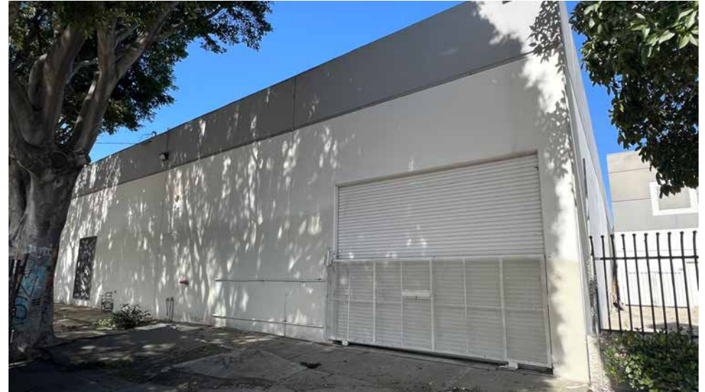
Ground Level Loading
