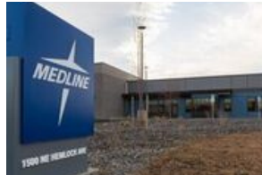
Medline Renewal Building -Photo Courtesy: Tim Park
