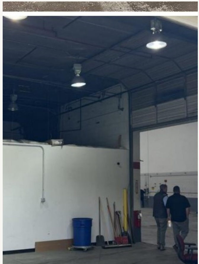
Oversized at-grade rollup door
