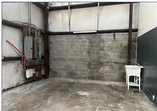
MOP SINK / UTILITY AREA
