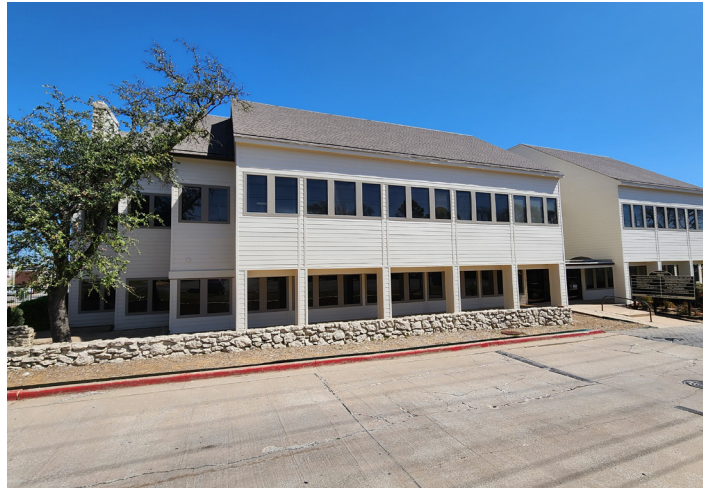
Side of Building Exterior
