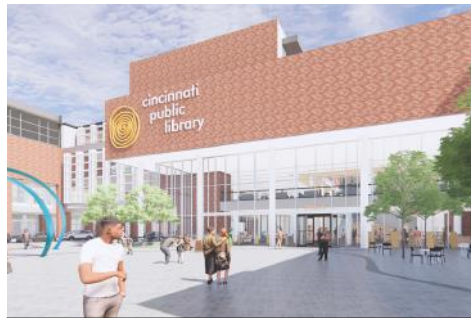
Public Library Renovation Major Renovation of Public Library
