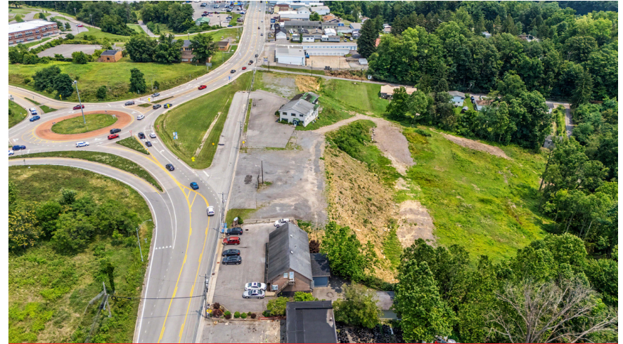
Aerial View Mileground Roundabout
