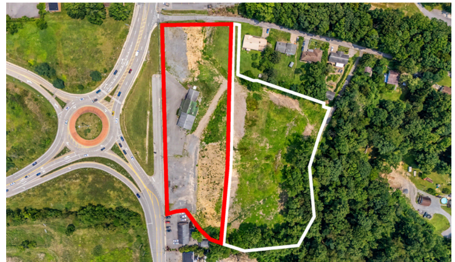
Aerial View Mileground Roundabout
