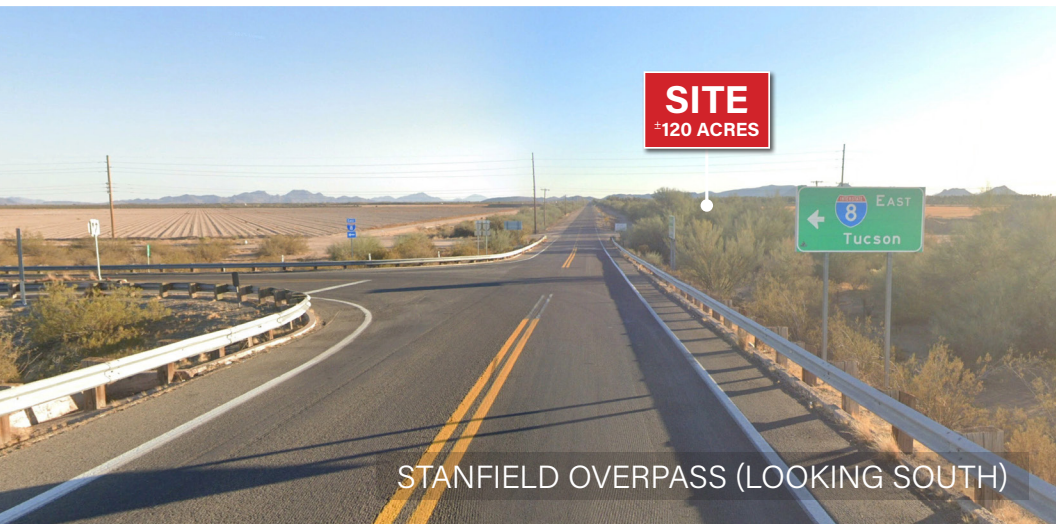
EAST ENTRY OF SITE (LOOKING WEST)
