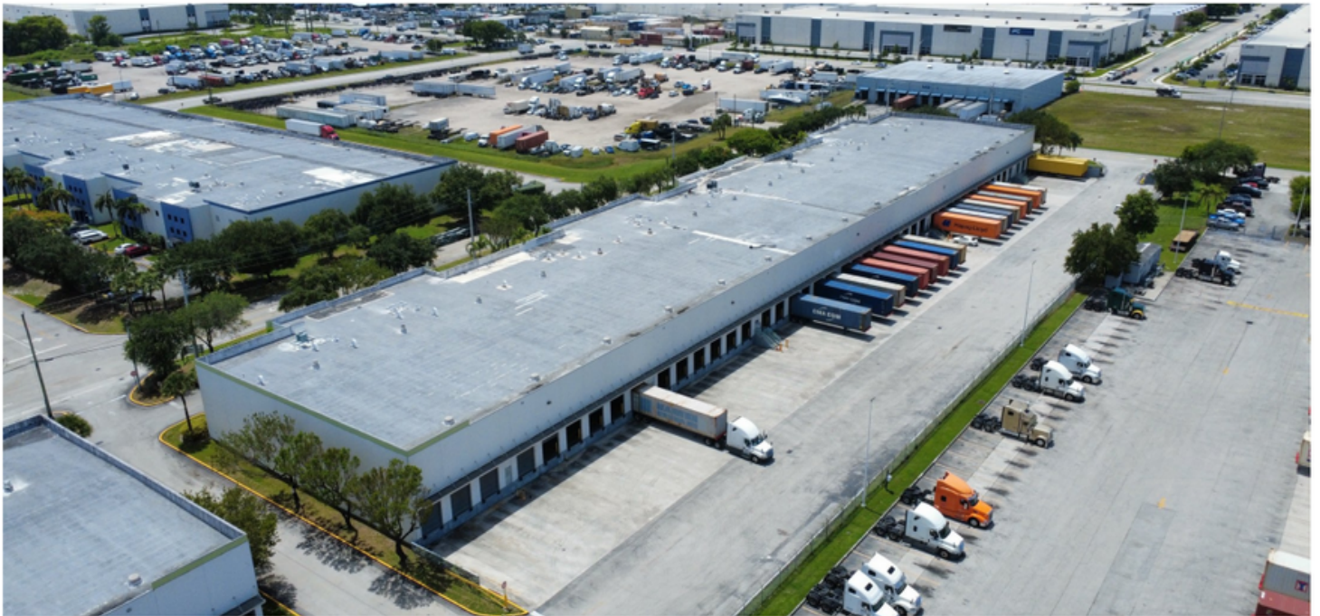
Aerial view of dock-high loading and private truck court along the rear of the Building.
