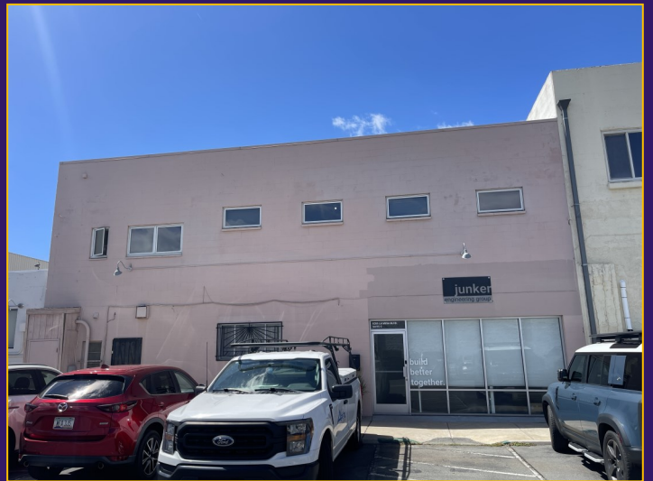
Outside with view of windows upstairs
