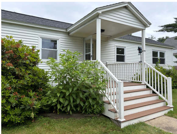
Renovated unit — entrance and deck
