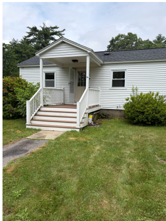
Renovated unit — front exterior
