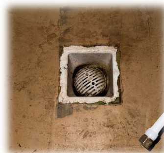
Floor drain for sink
