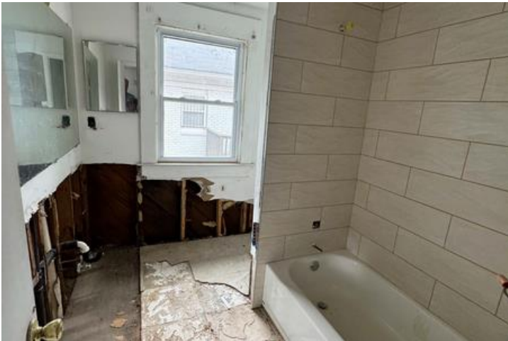
Left: bathroom — shower tile complete, fixtures and vanity pending.
