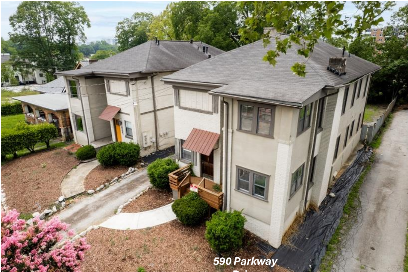
590 Parkway Drive NE - secured while renovation work is in progress.
