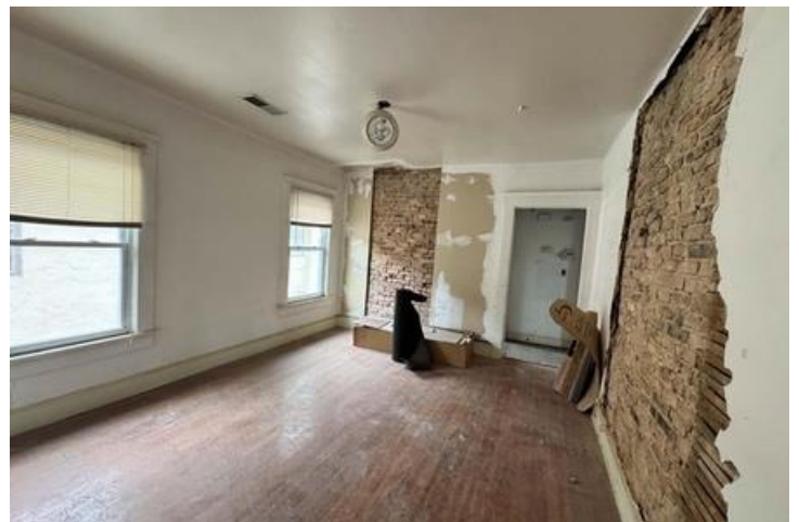
Right: original brick masonry exposed during framing work.
