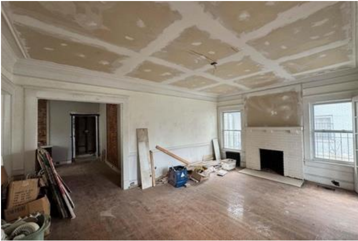
Left: living room — ceiling and trim work complete, original fireplace intact, awaiting paint.
