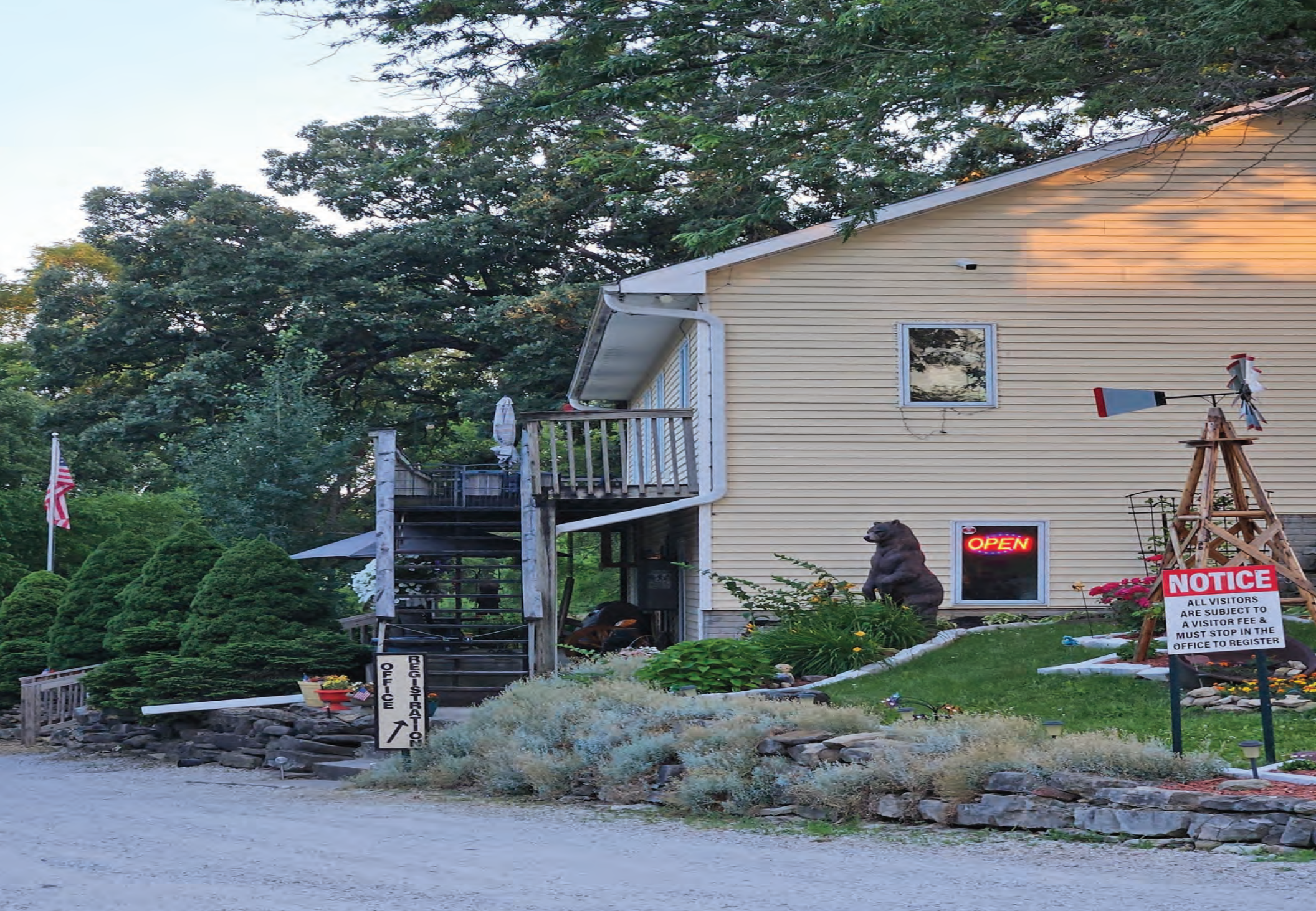
Lodge (top level = living quarters, lower level = office)
