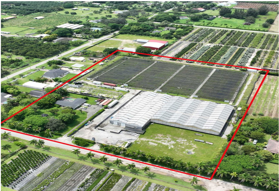
Aerial view — 6.10-acre nursery parcel outlined
