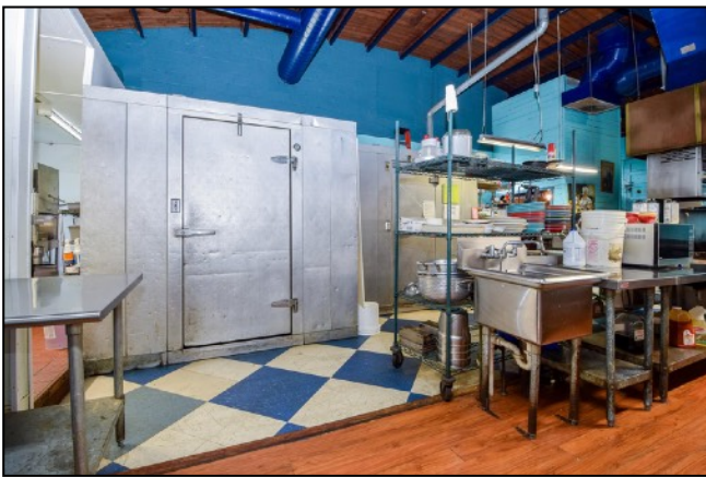
Main Level Walk-In Freezer & Refrigerator
