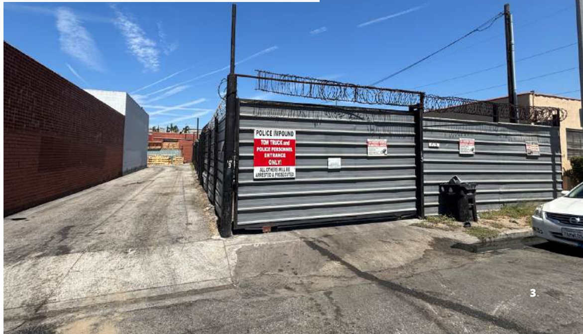
View of 715 Vesta St. Yard Looking North from Vesta St.
