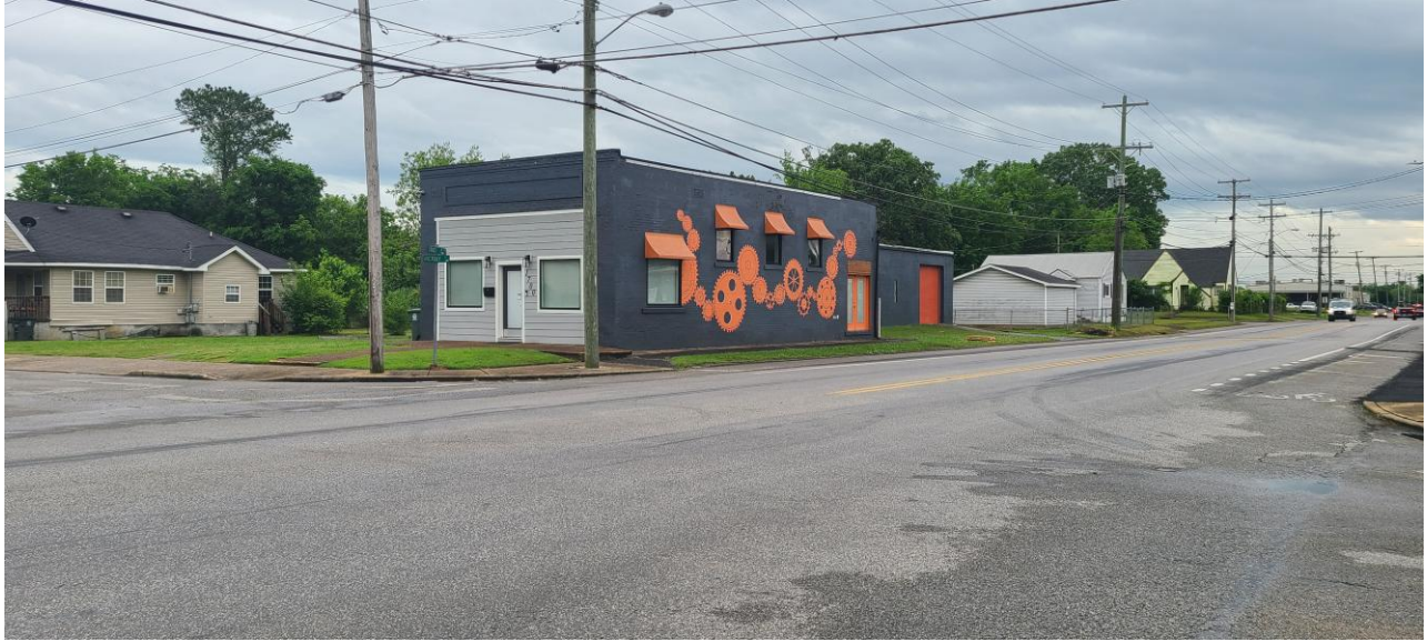
Corner of Foust Street and South Hickory Street
