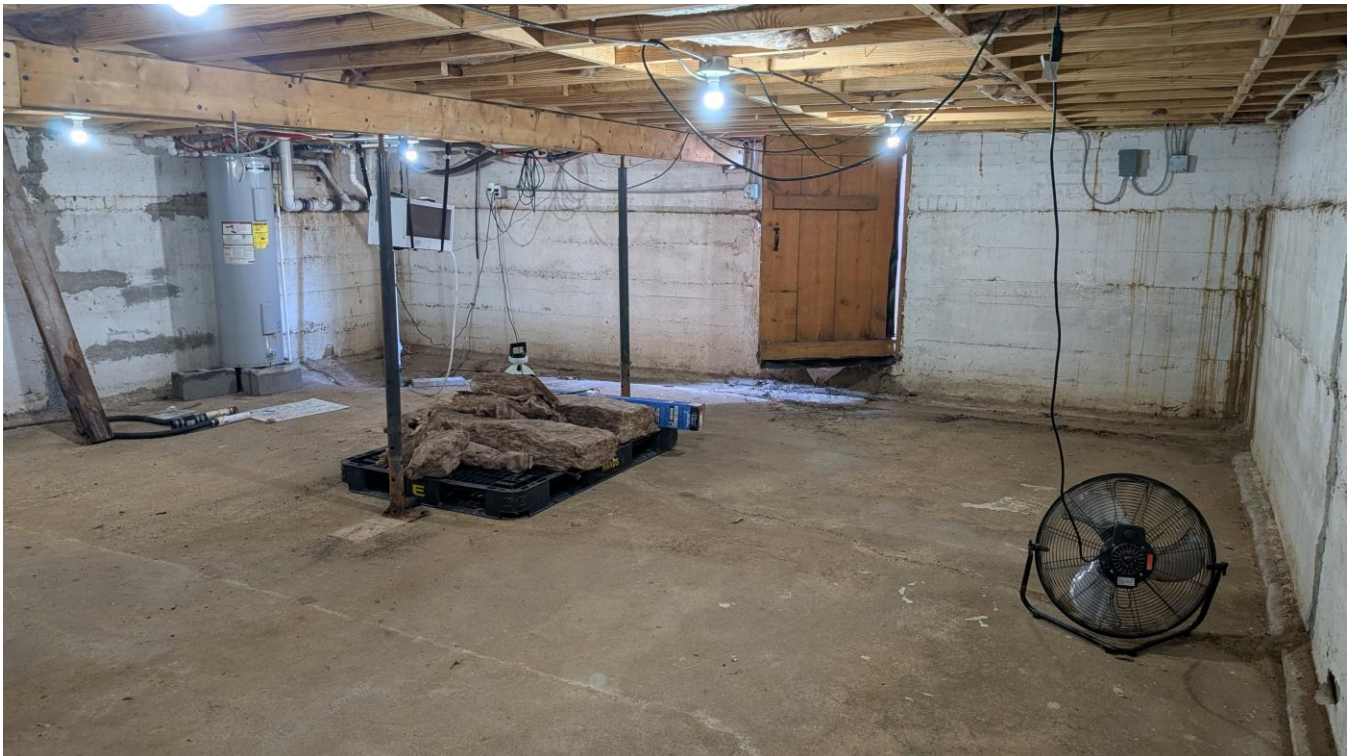
Exterior basement access
