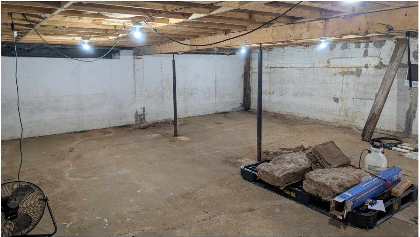
Basement sits under a portion of the front office area
