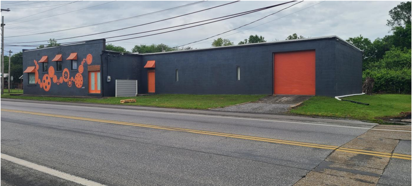
Additional exterior doors: Double-doors to office, single door to warehouse, roll-up door to warehouse
