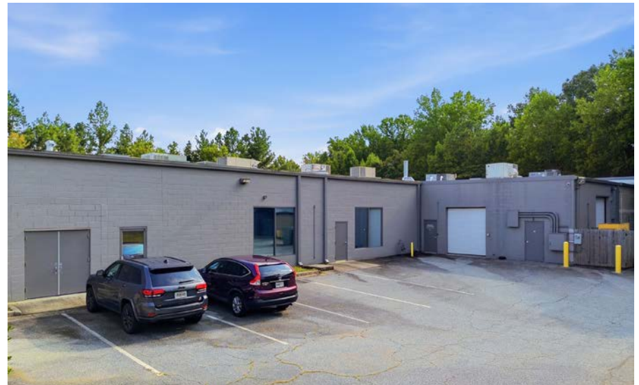
Rear service elevation - rooftop units, roll-up doors and screened utility yard
