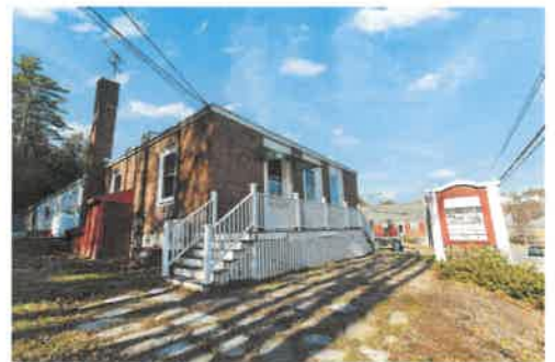
Front Entry and Window Service Deck
