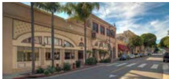
BROWN BROTHERS BUILDING San Pedro
