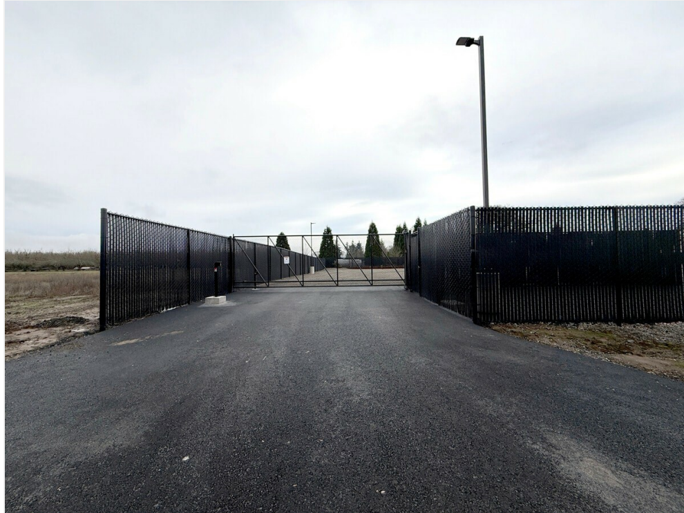
Access Gate - 20 Feet Wide
