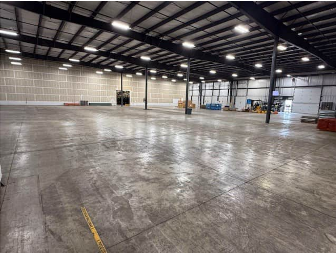
SE CORNER LOOKING NW
