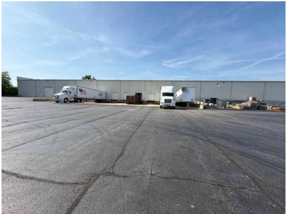
DOCKS NORTH/REAR SIDE
