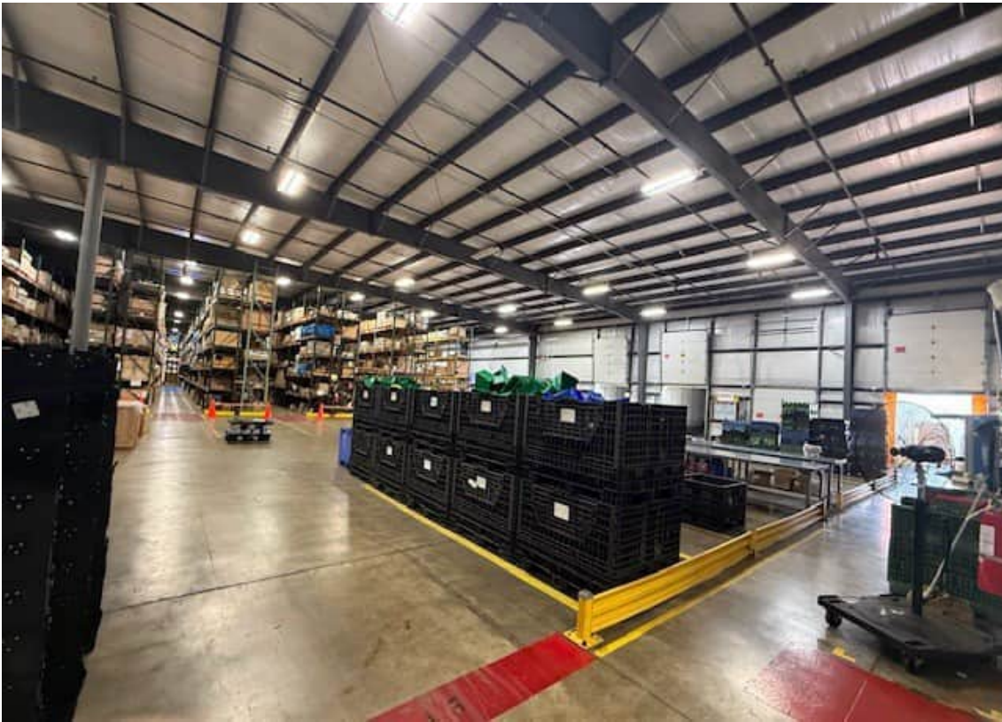
OPENING IN DEMISING WALL LOOKING TOWARD DOCKS
