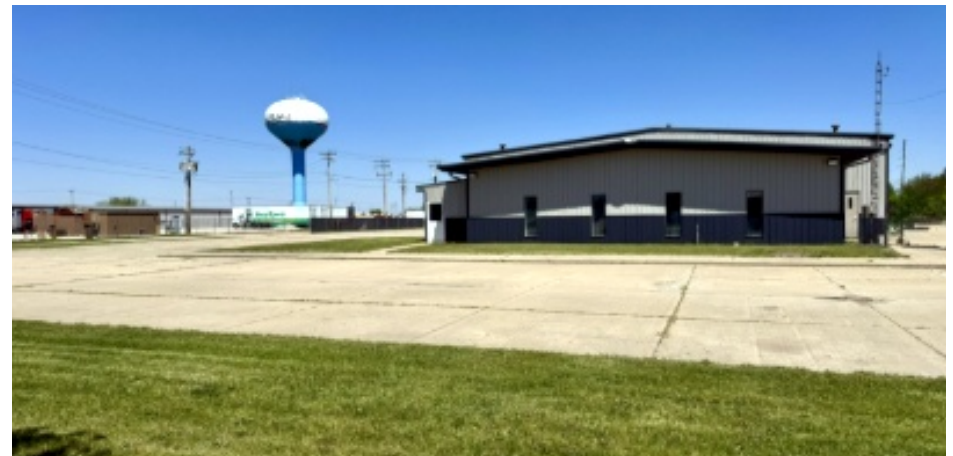
Side Exterior and Yard Area
