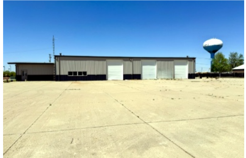
Multiple Overhead Doors with Large Concrete Yard
