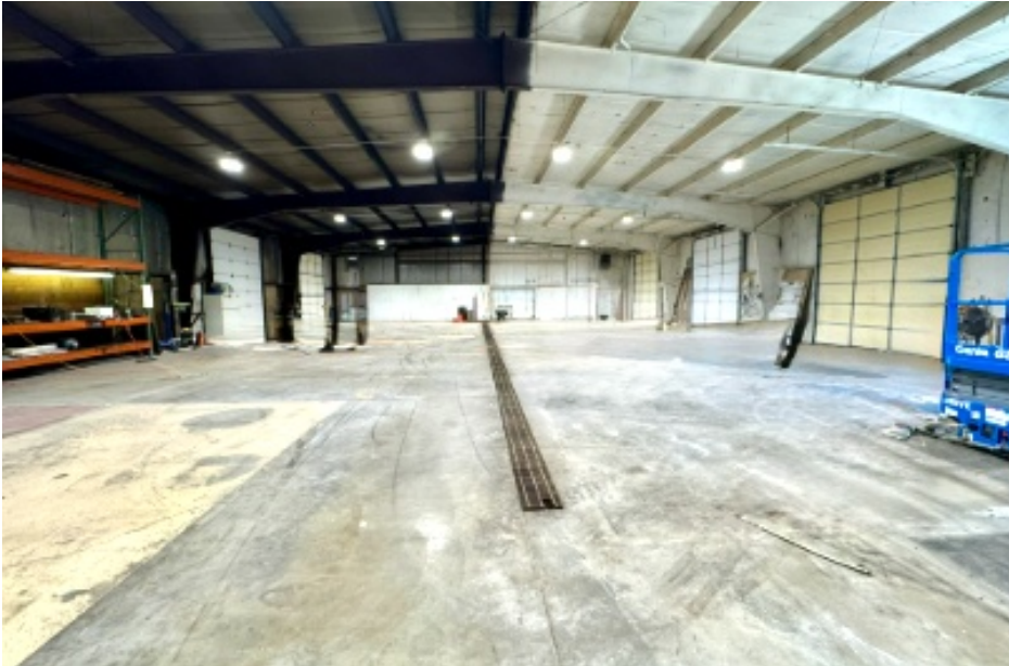
Large Industrial Shop with Floor Drain
