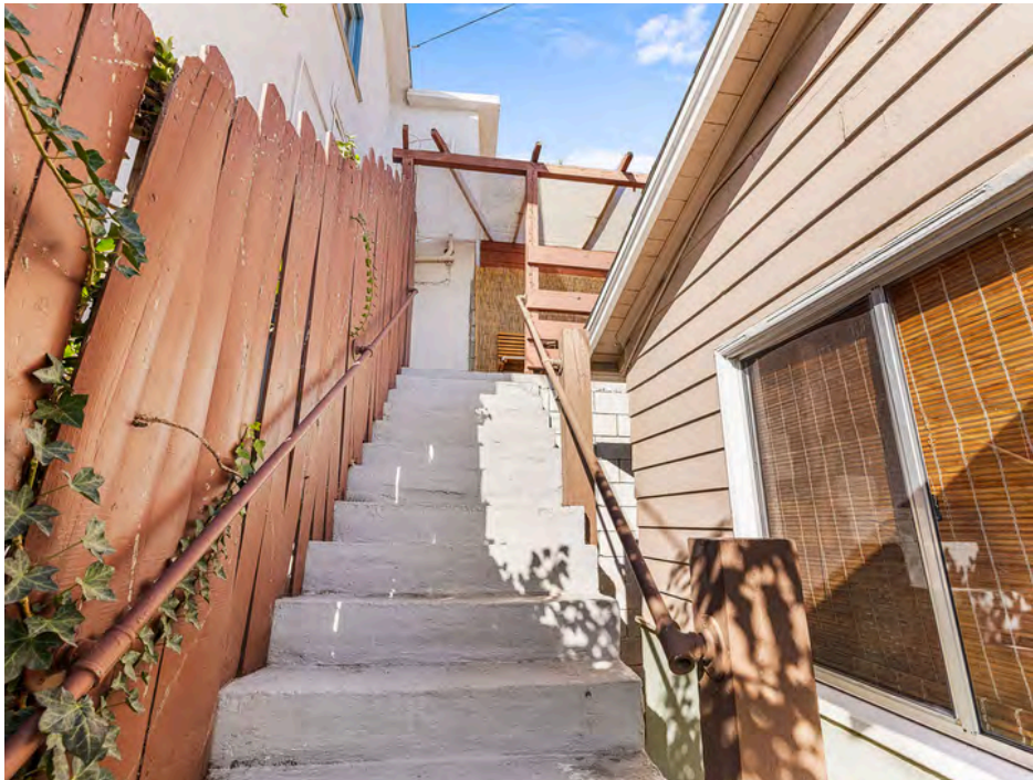
Stairs Leading from Unit 3053 to Upper Property Entrance
