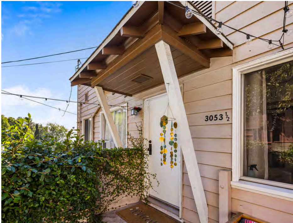
Entrance to Upper Unit 3053 1/2
