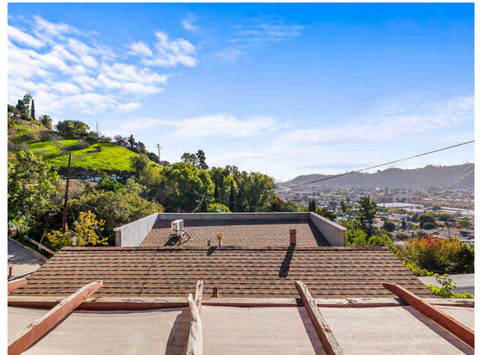
View From Roof Facing South
