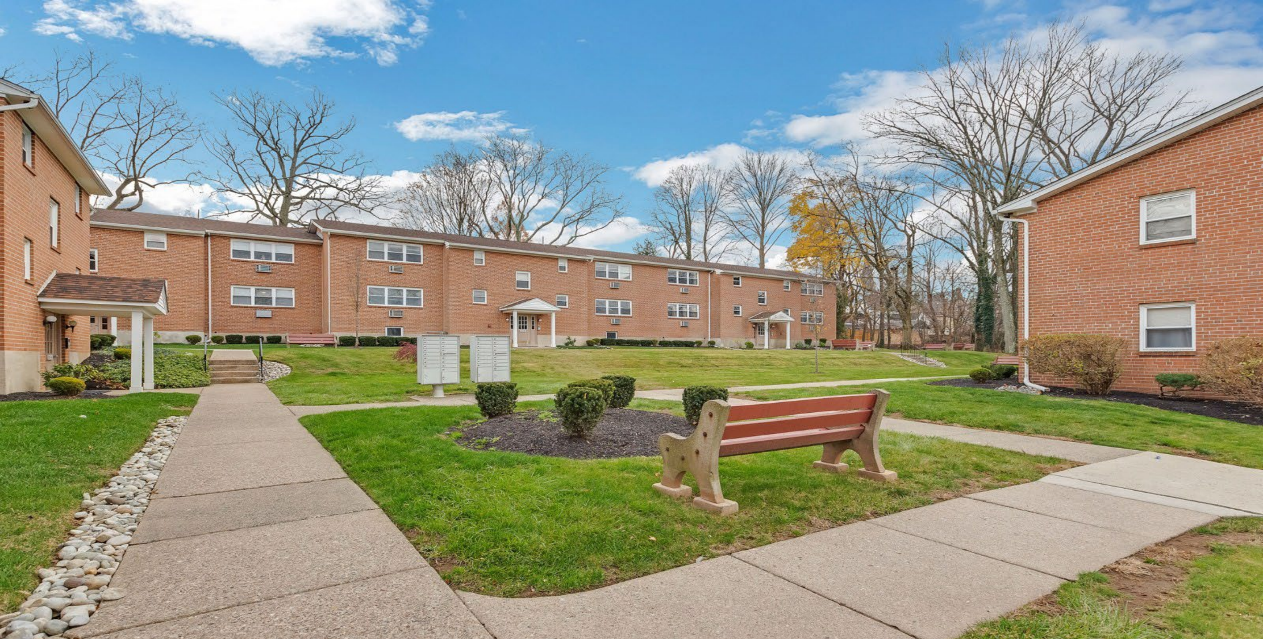
EXTERIOR · SPRUCE COURT APARTMENTS
