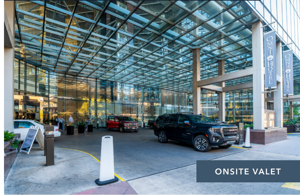
NO CIRCLING. JUST CURBSIDE CLASS FOR CLIENTS
