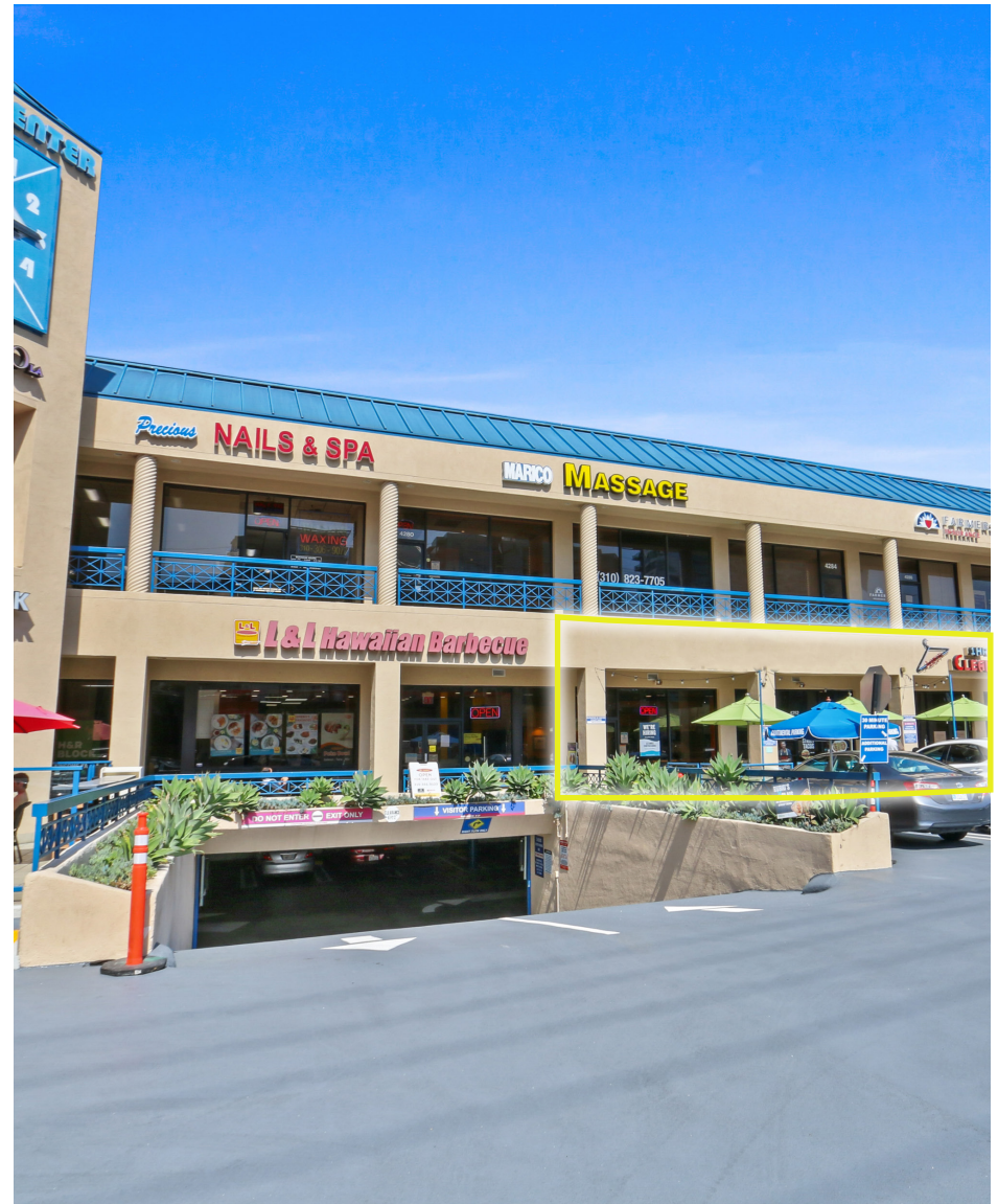
Entrance to subterranean parking
