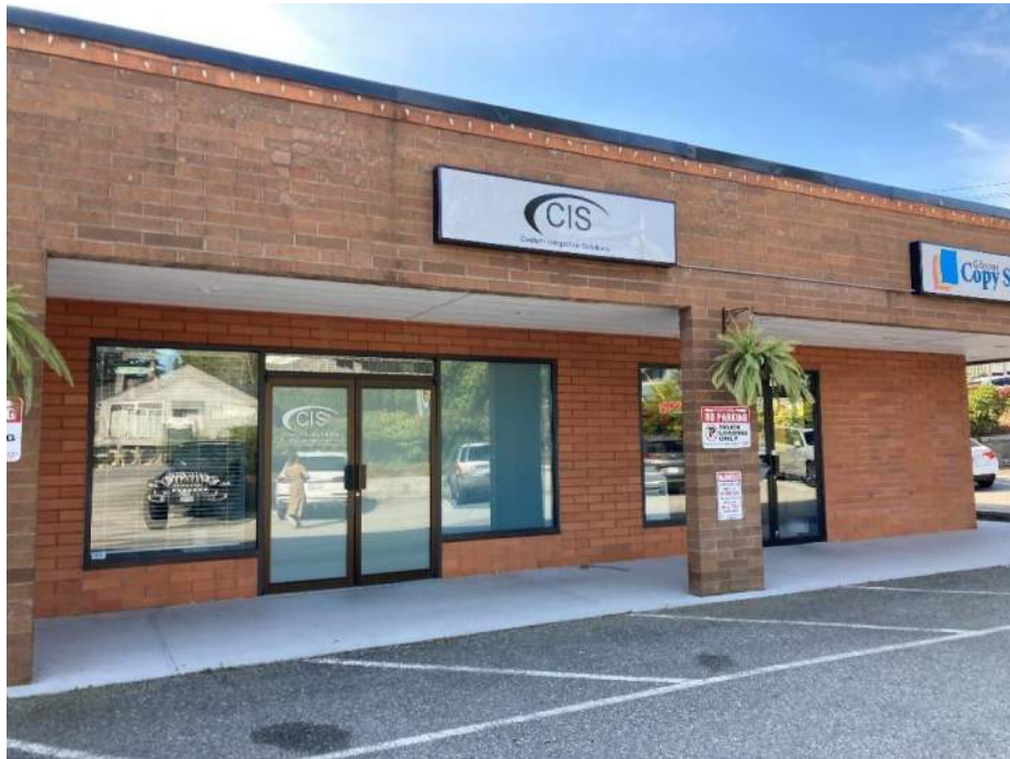
Photograph No. 18. View of Unit 5 – CIS: Custom Integrated Solutions.
