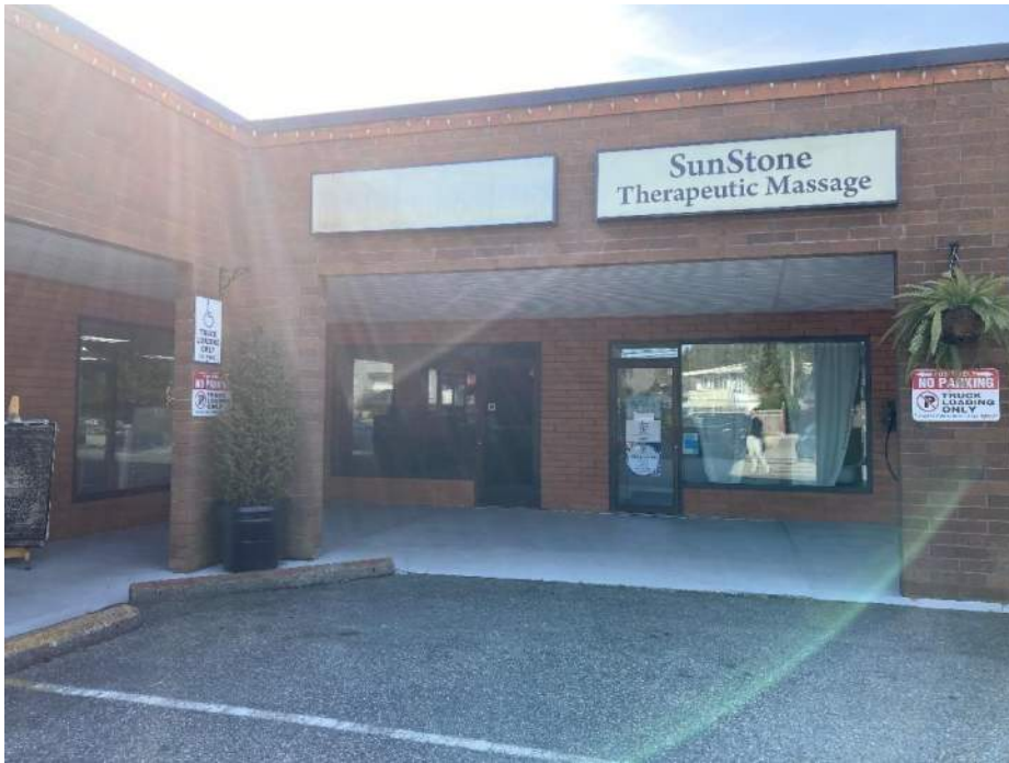
Photograph No. 12. View of Units 2 (Vacant) and 3 (SunStone Therapeutic Massage).
