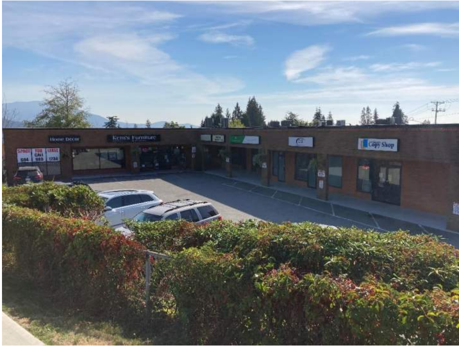
Photograph No. 1. Site building; photograph taken facing east from School Road.
