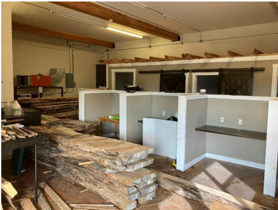
Photograph No. 26. View inside Unit 10 – vacant office space currently used as storage for the building owners at the time of the Site visit.
