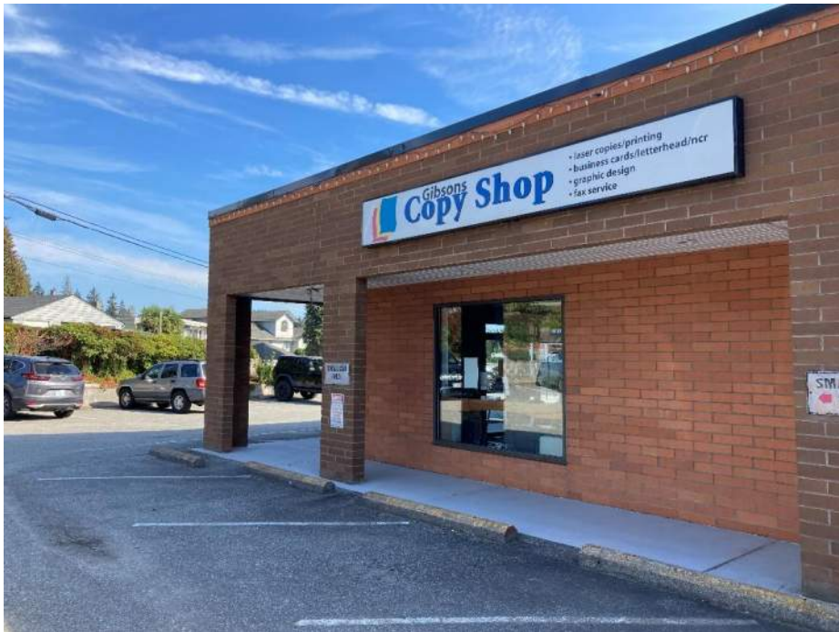
Photograph No. 20. View of Unit 6 – Gibson's Copy Shop.
