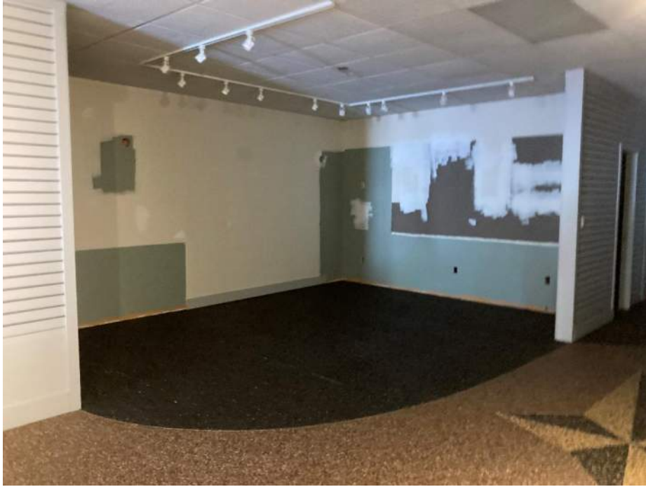
Photograph No. 13. View of vacant space within Unit 2.
