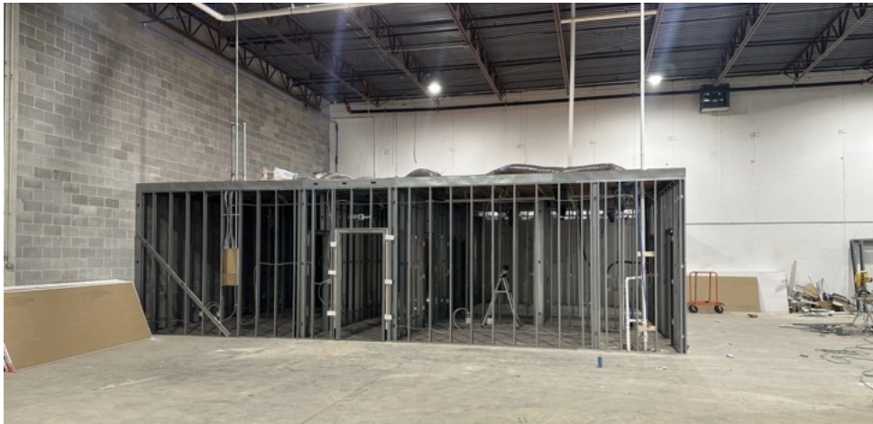
Framed office space that will have 3 offices, 2 restrooms and conference room
