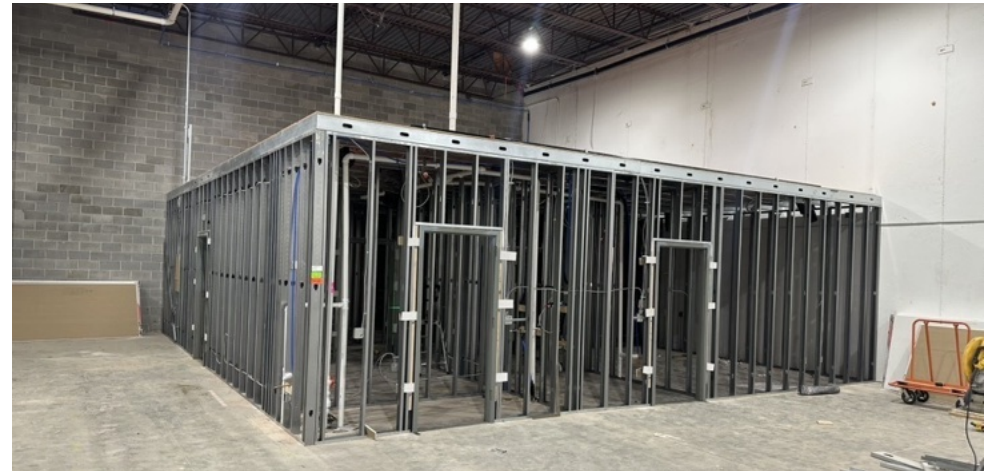
Another view of the newly framed office space
