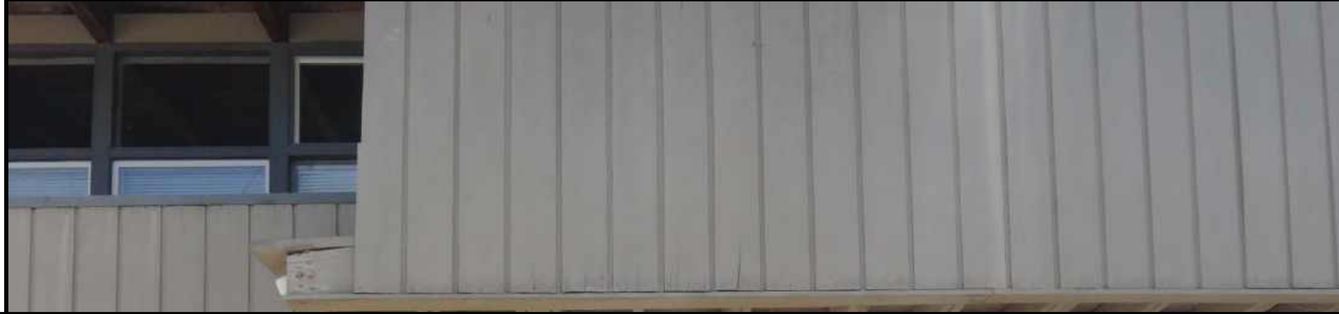
4 PROJECT AS-IS PHOTO
