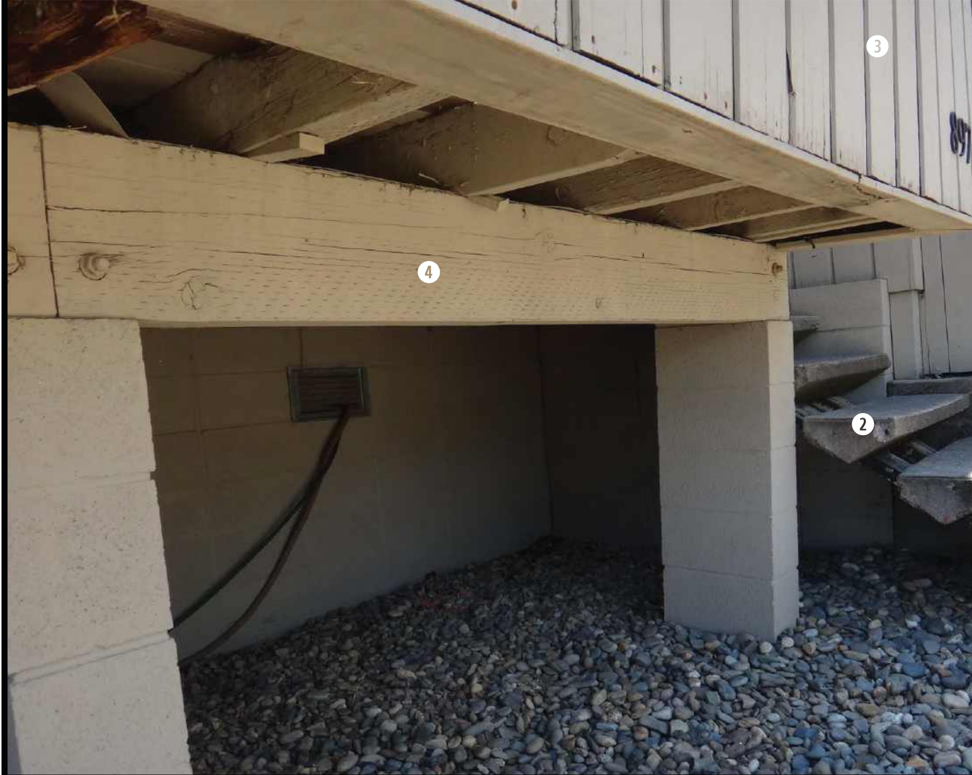
4 PROJECT AS-IS PHOTO
