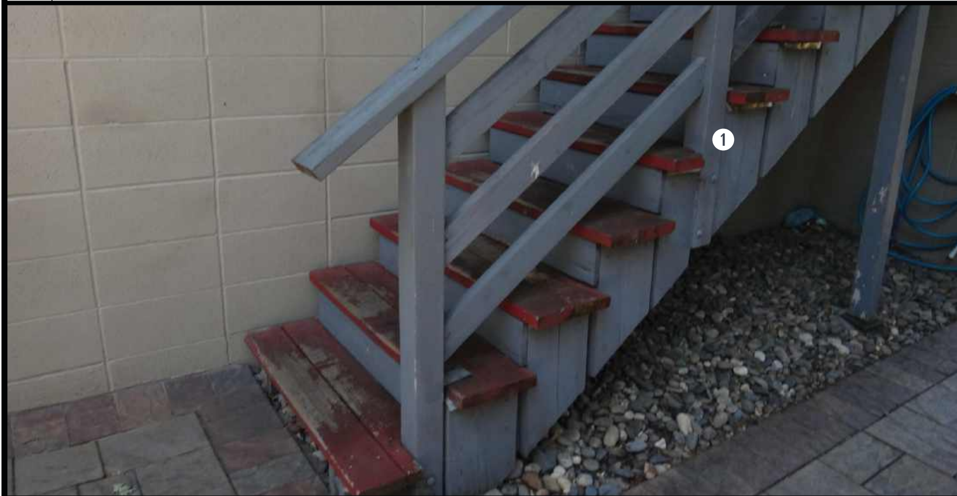
4 PROJECT AS-IS PHOTO
