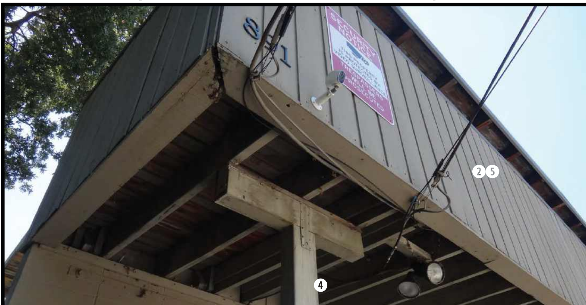
6 PROJECT AS-IS PHOTO
