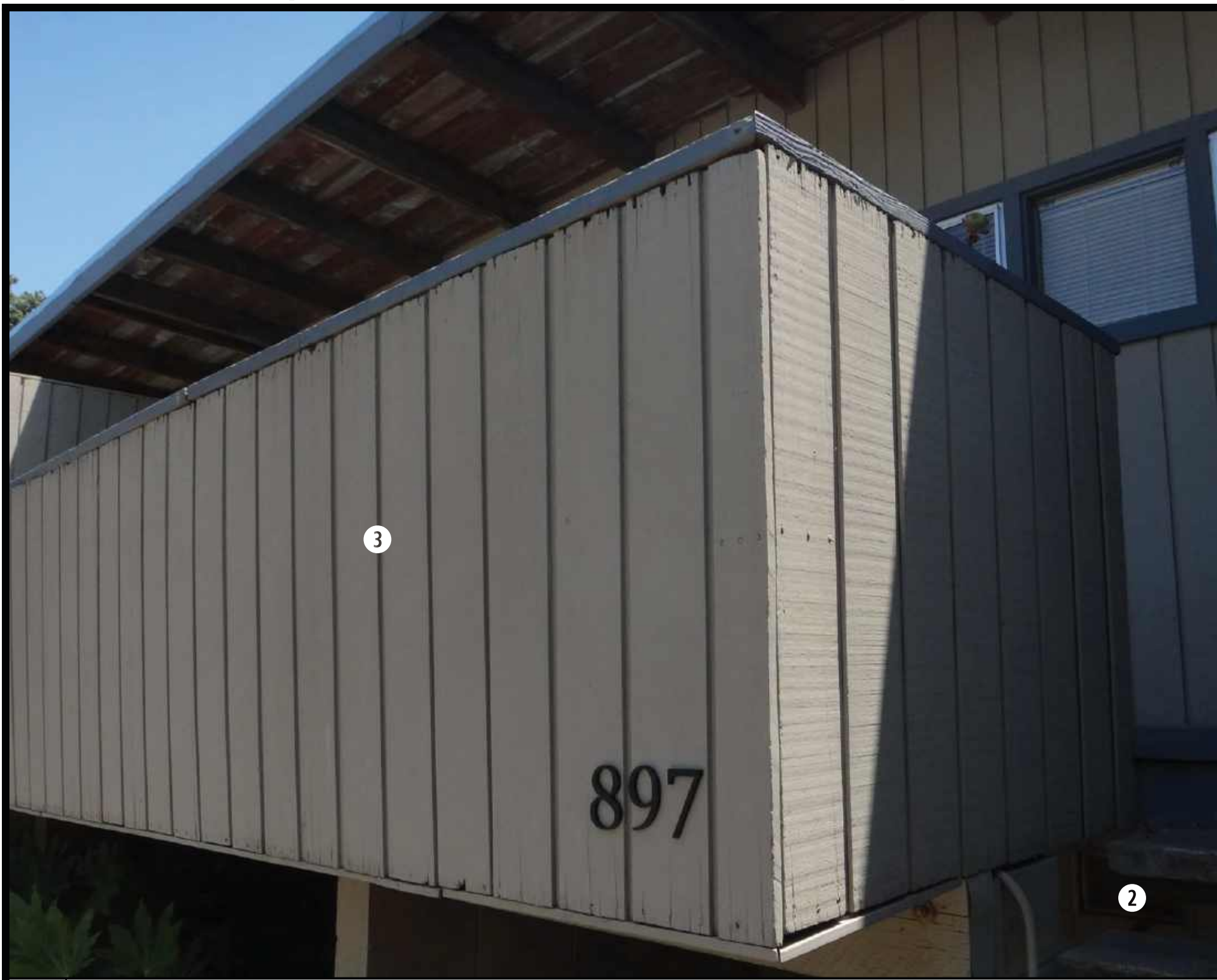
5 PROJECT AS-IS PHOTO
