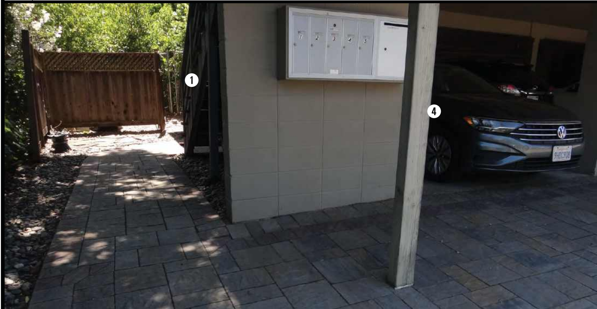
5 PROJECT AS-IS PHOTO
