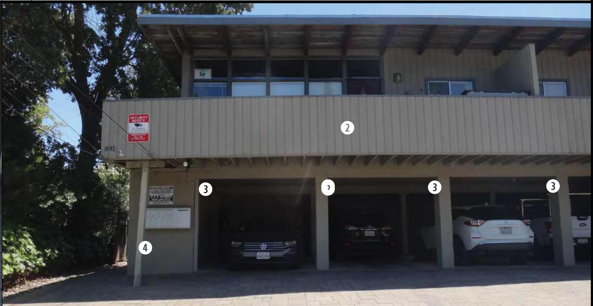
2 PROJECT AS-IS PHOTO
