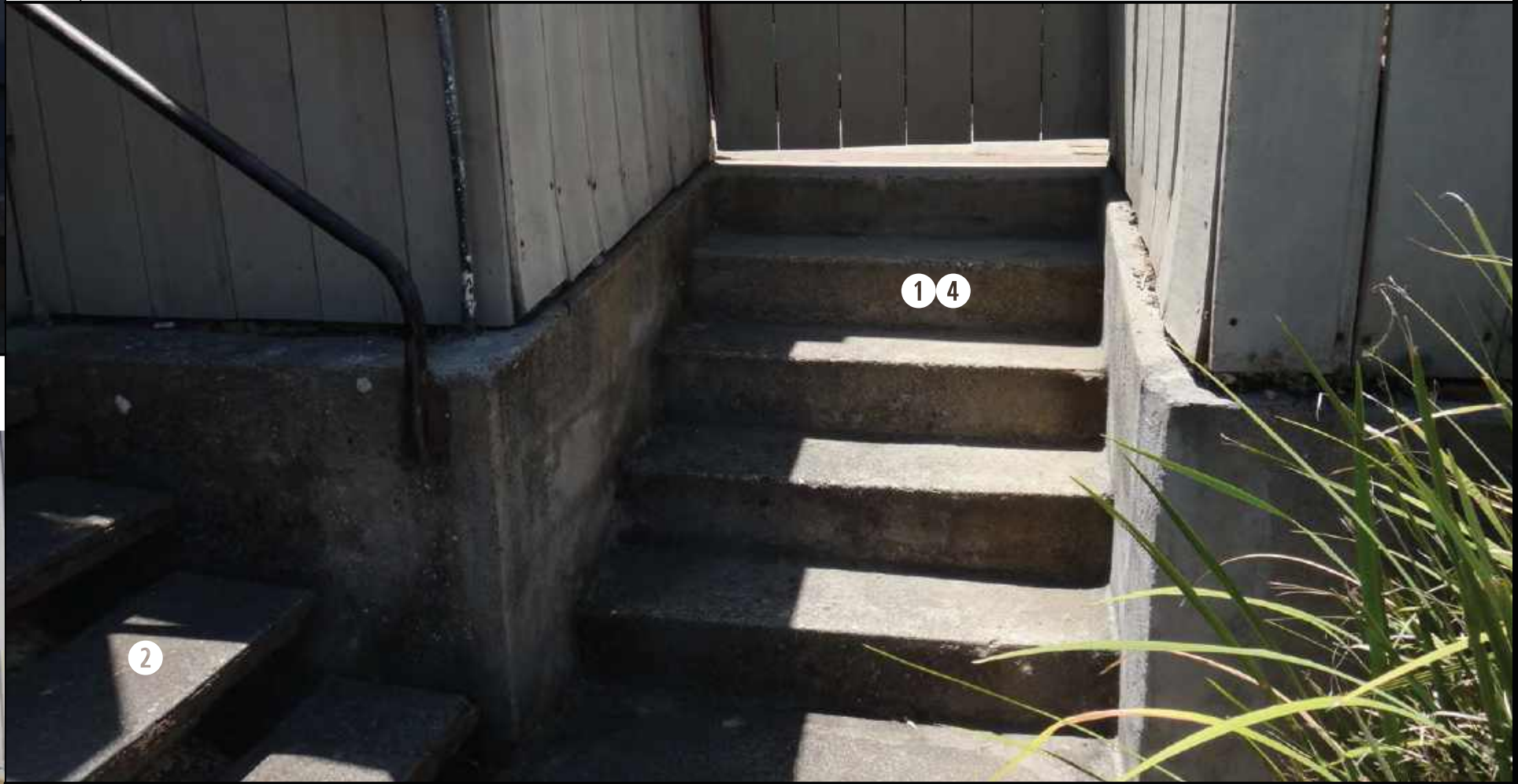
2 PROJECT AS-IS PHOTO
