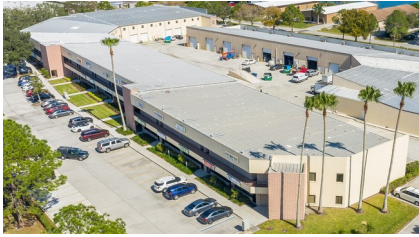
Aerial / Building View
