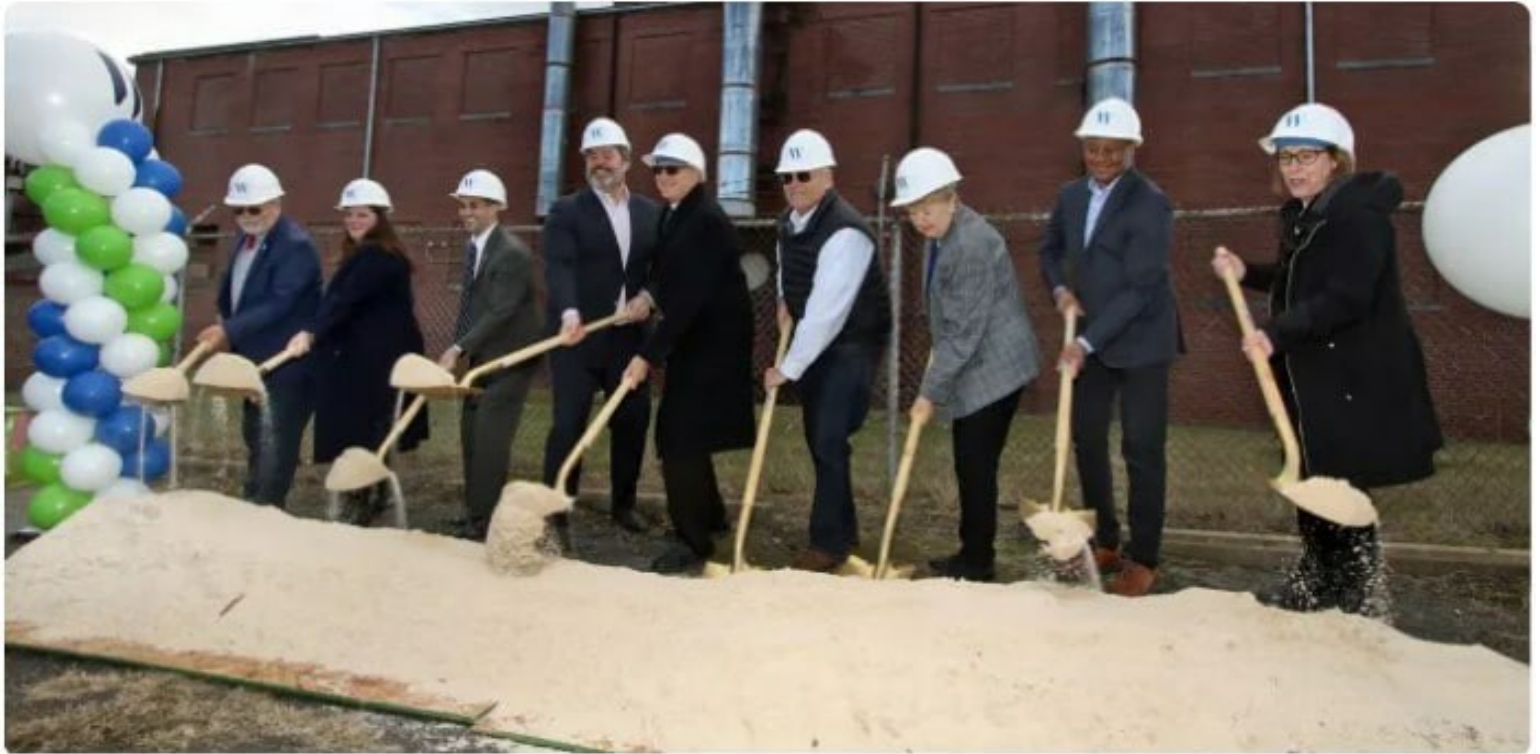
Dirt is shoveled during a ground breaking ceremony held on the grounds of Osage Mill in Bessemer City Thursday afternoon, Jan. 26, 2023.
