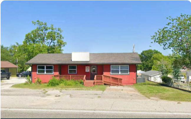
409 S Main St, Grove, OK 74344
