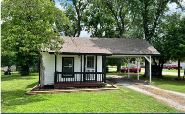
1007 S Main St, Grove, OK 74344
