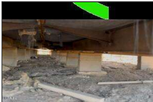
Piers Concrete Blocks under Mobile Home
