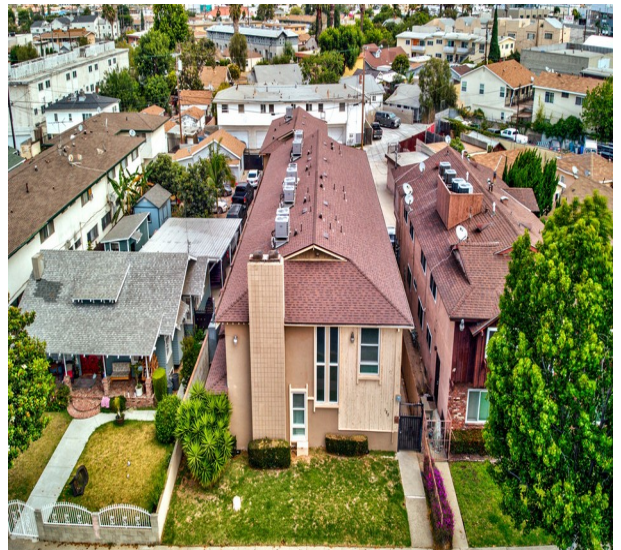
Front north-facing exterior
