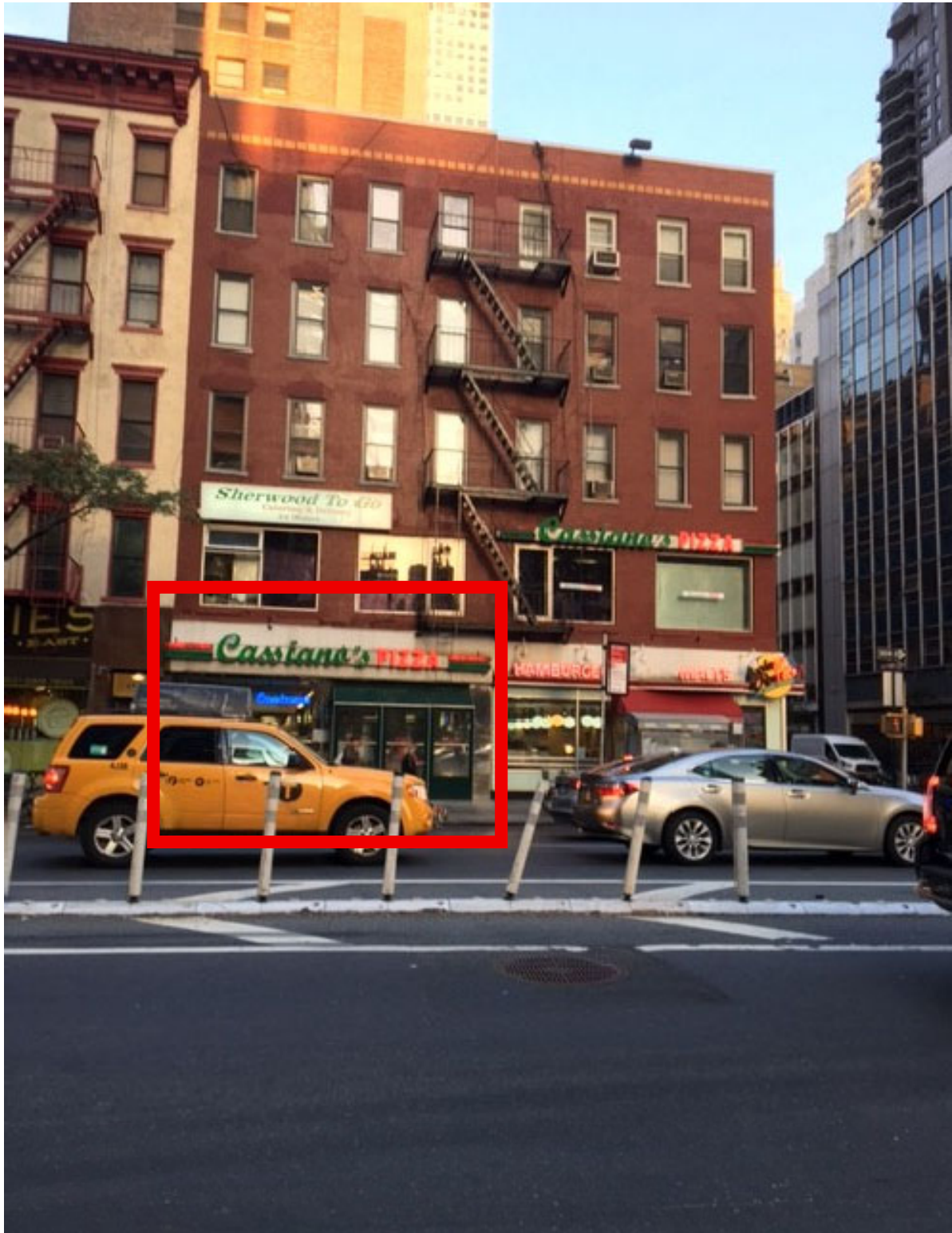
GROUND FLOOR SPACE ALONG 3RD AVE
