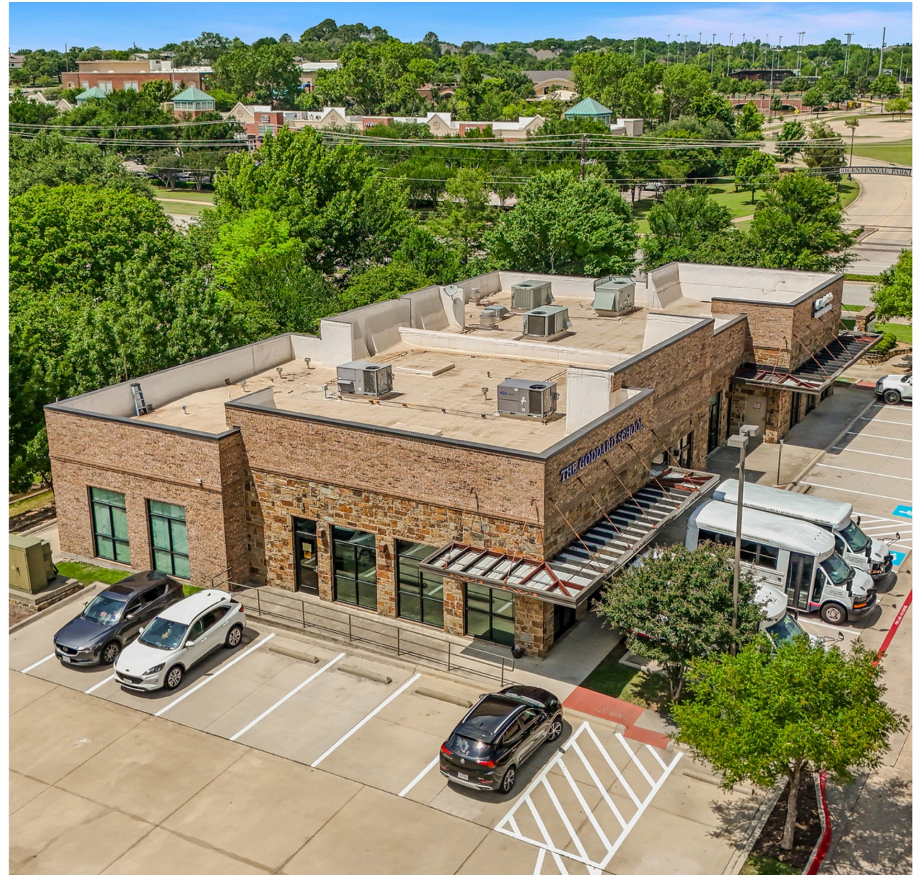
EXTERIOR · 445 W SOUTHLAKE BLVD
