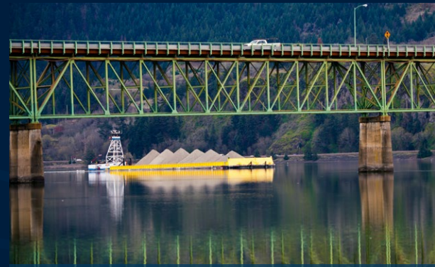
Direct Marine Access via Deepwater Docks
