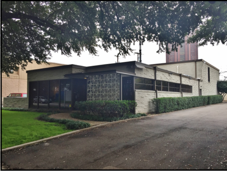
Front of Building
