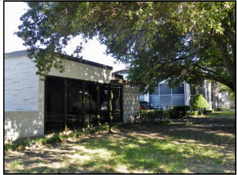
Front of Building
