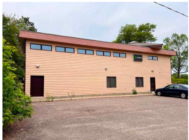
Back Side of Building
