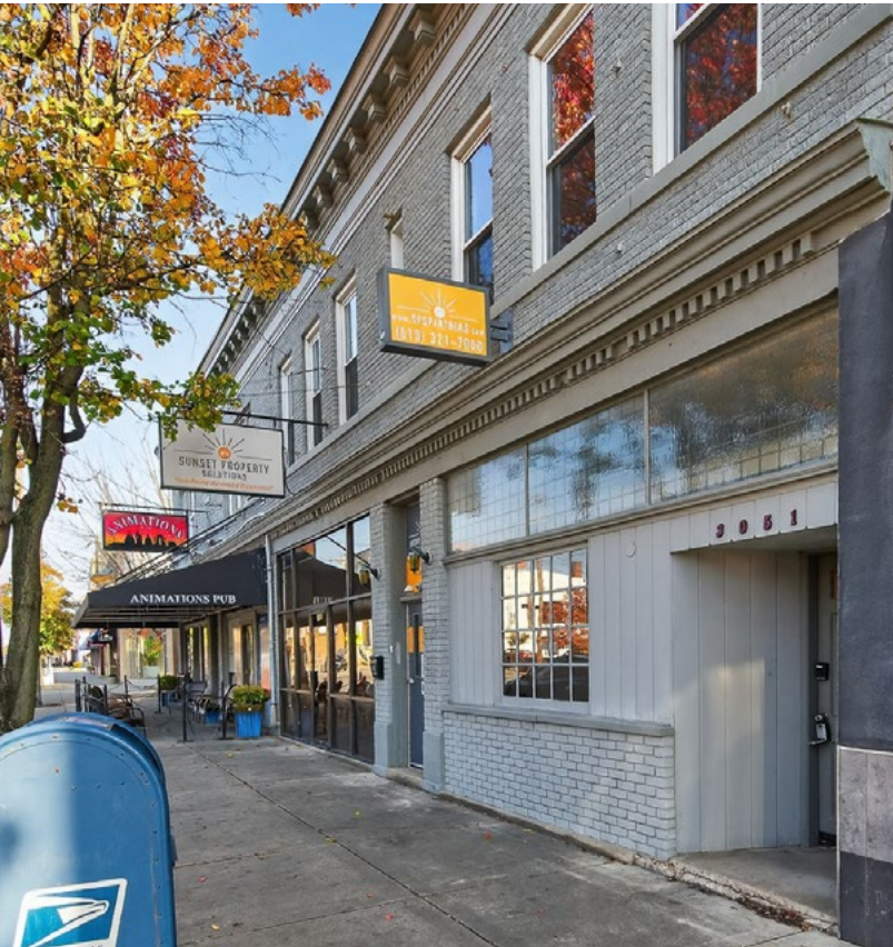
Building Entrance (SW Angle)
