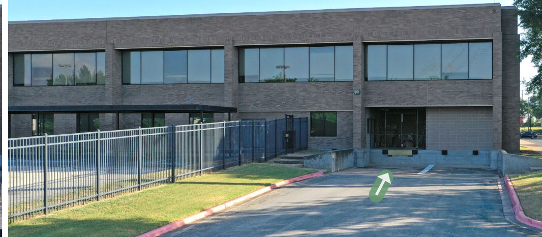
Reinforced Loading Dock (east wing)
